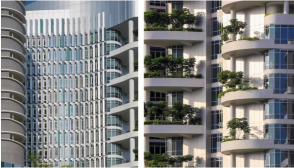
Fig. 11. Use of sunscreen in a hospital complex Ng Teng Fong (NTFGH) & Jurong (JCH).
