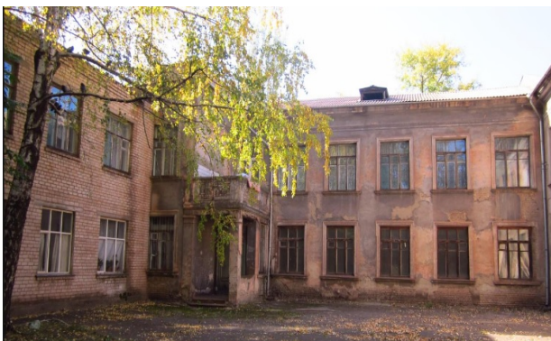
Fig. 4. Hospital building No.3, Kryvyi Rih.
