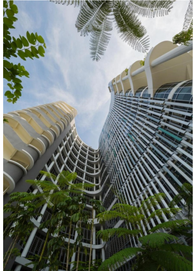
Fig.10. Exterior of hospital complex Ng Teng Fong (NTFGH) & Jurong (JCH).
