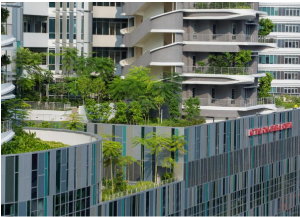
Fig. 16. Implementation of green roofs.
