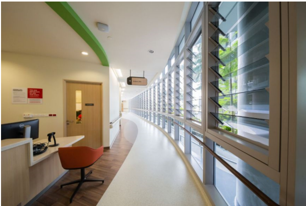
Fig. 12. Sun blinds in hospitals interior Ng Teng Fong (NTFGH) & Jurong (JCH).
