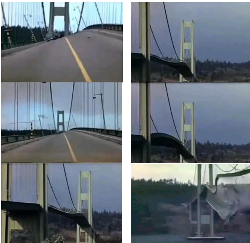
Fig. 4. Tacoma Narrows Bridge collapse “Galloping Gertie” November 7, 1940.
