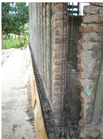
Fig. 12. Repair and retrofitting of non-engineered building by adding the reinforcement of tie beams, columns and link-beam
