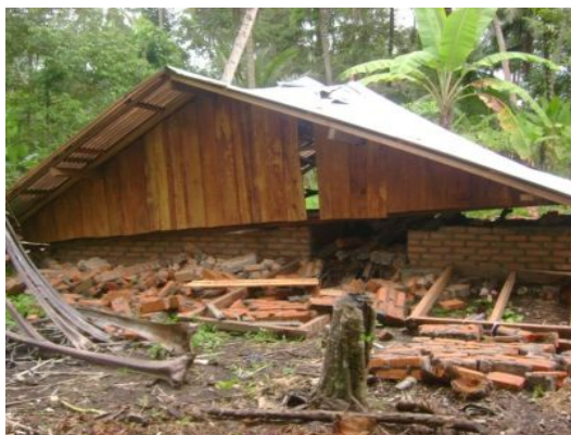
Fig 6. Brick walls collapsed
