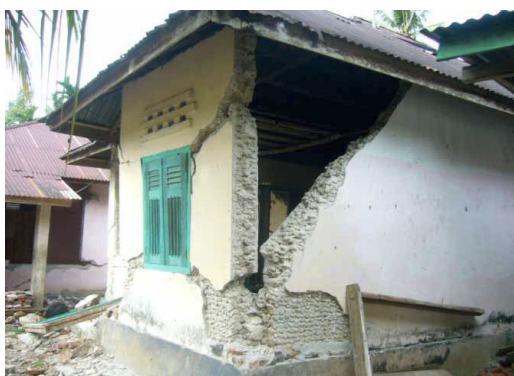
Fig 7. Wall separation of URM
