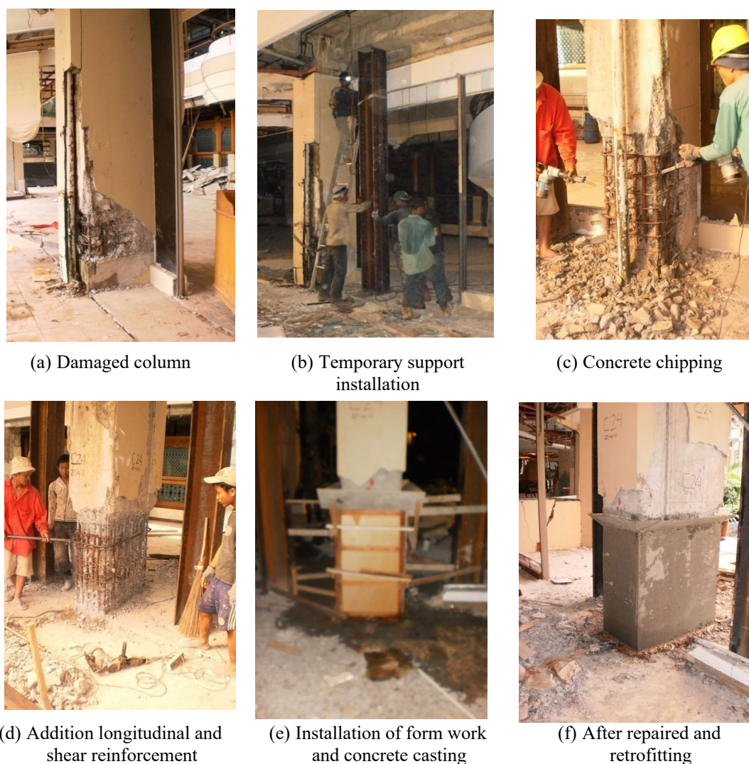
Fig. 9. Repair and retrofitting process of damaged column at the bottom.
