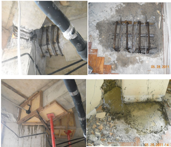
Fig. 11. Repair and retrofitting process of damaged beams
