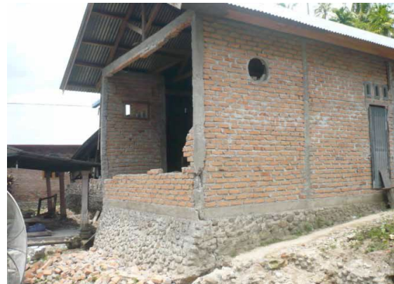
Fig 8. Some brick walls are collapsed
