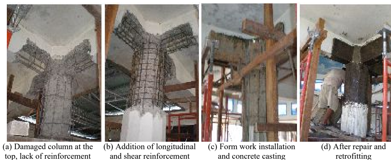
Fig. 10. Repair and retrofitting process of damaged column at the top.
