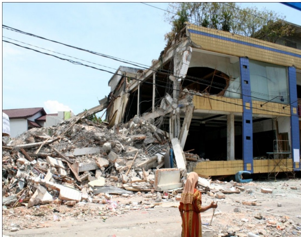
Fig 5. Building collapsed due to material quality do not meet the standards
