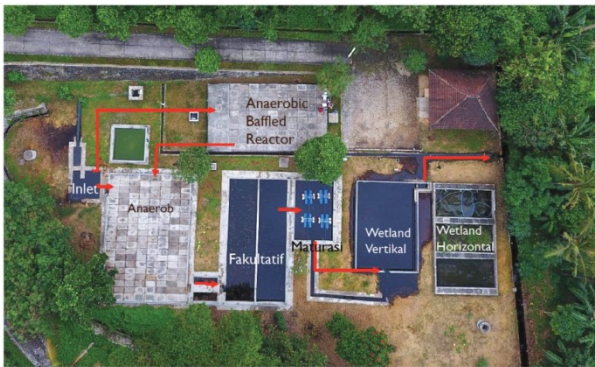
Fig.1. Leachate treatment plant aerial view in Temesi landfill [12]
