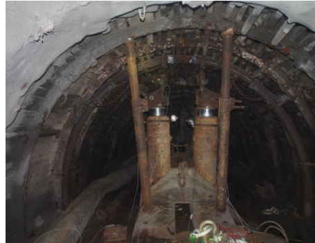
Fig. 18. Testing equipment ready to use installed in testing site (photo P.Ficek).
