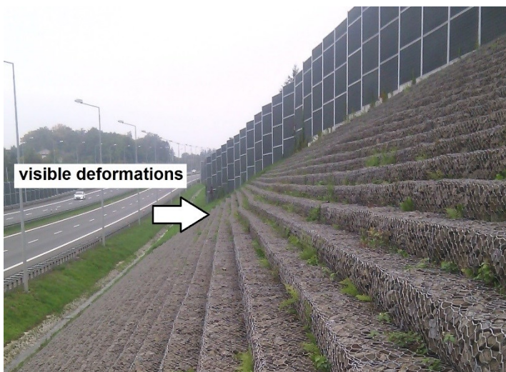
Fig. 9. Overview of the slope with retaining structure and the noise barriers (photo by authors).
