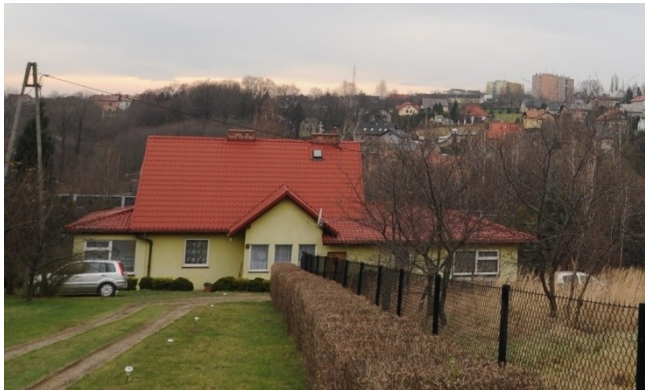
Fig. 7. The house located on the slope in the analysed case (photo by authors).
