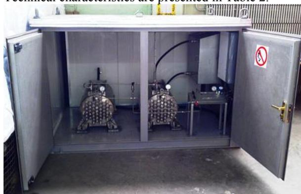
**Fig.9.** Long-term stationary metal hydride hydrogen storage system for backup power supply.
