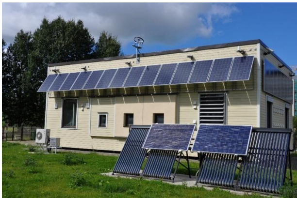
Fig. 1. Tallinn University of Technology nZEB test facility [7].
