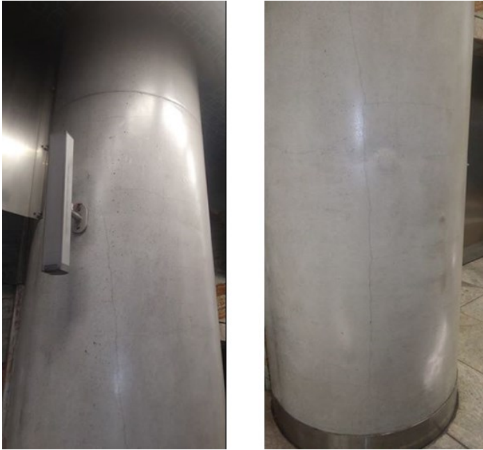
Fig. 3 View of scratches on a single pillar
