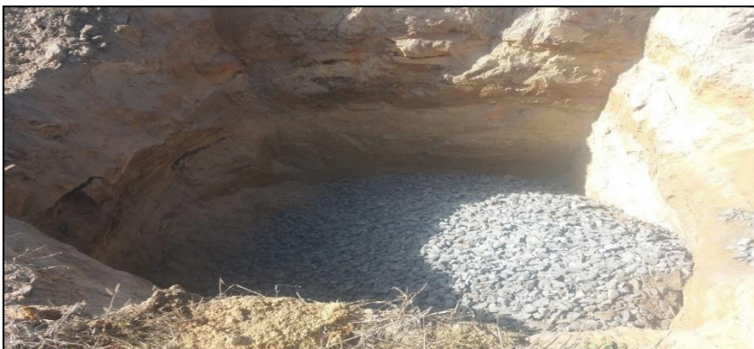
Fig. 10. The filling of the landslide located in the area of the Lubichów IVa shaft.
