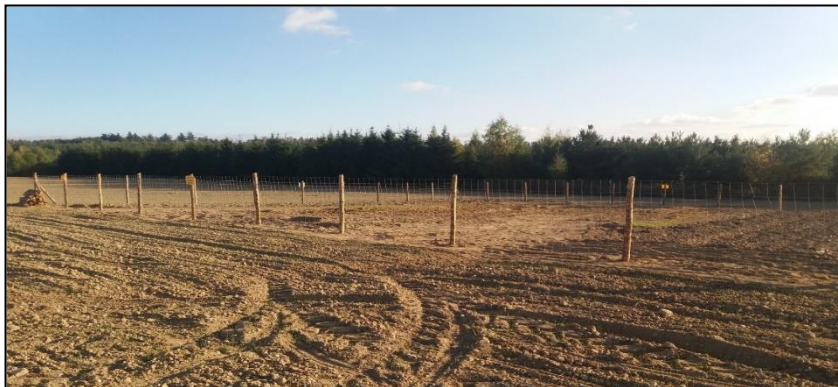
Fig. 11. The fence around the area of the landslide under surveillance.
