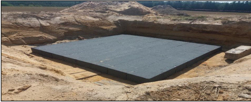
Fig. 7. Reinforced concrete slab approx. 3m under terrain level, dimensions: 7.0x7.0x0.5m
