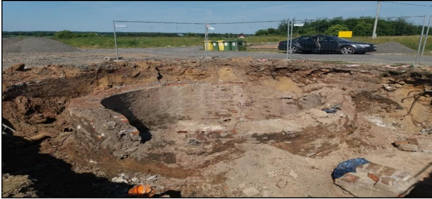
Fig. 4. Exposed Lubichów III shaft barrel.
