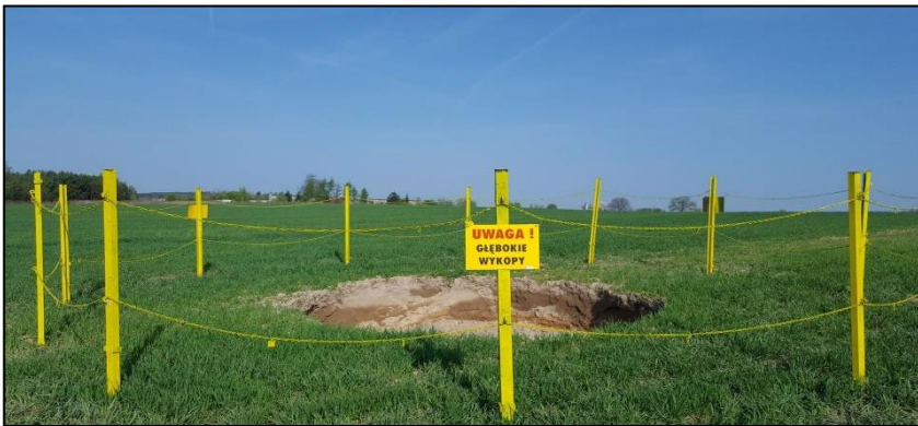
Fig. 9. Secured sinkhole in Lubichów IVa shaft area.
