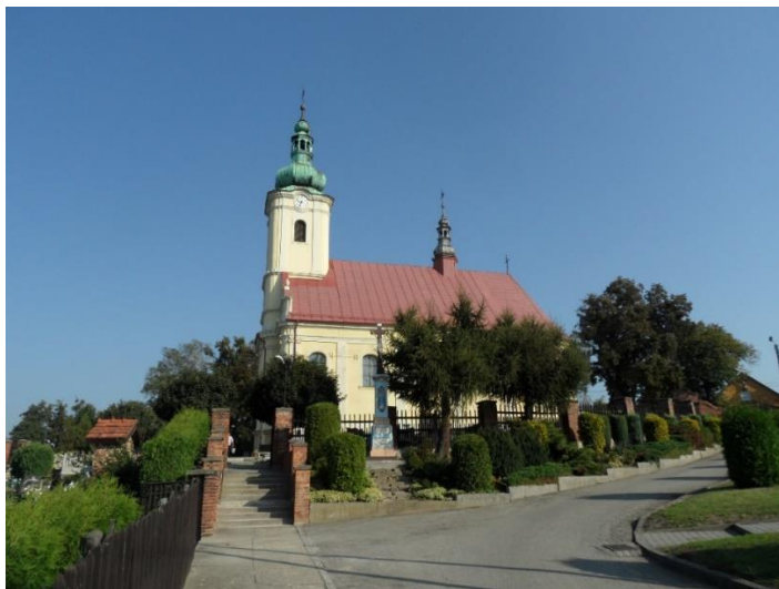
Fig. 1. General view of the church building.
