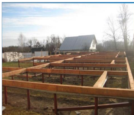
Fig. 8. Screw pile foundation
