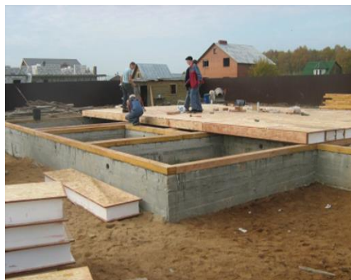
Fig. 7. Shallow foundation
