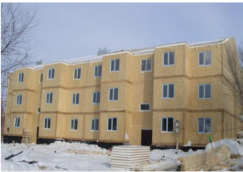
Fig. 2. Multi-familial residential house made of SIP-panels
