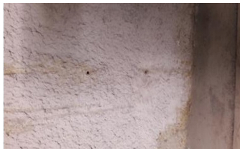
Fig. 2. Dampness in the connection between the diaphragm wall to the foundation slab
