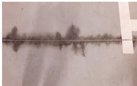
Fig. 3. Leaks in the floor over the foundation slab
