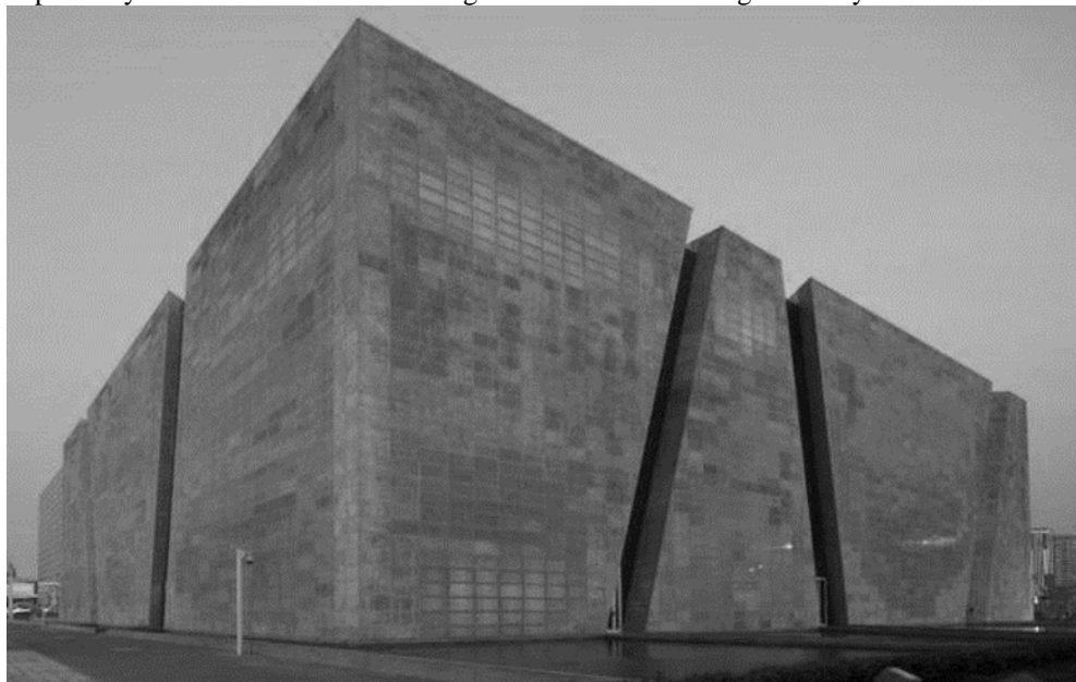
Fig. 8. Office building with walls of translucent concrete.
