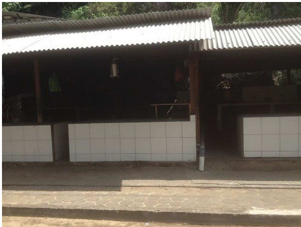
Fig. 5. Evacuation Route Signs (up); design of the shops that potentially delay the evacuation process (down).
