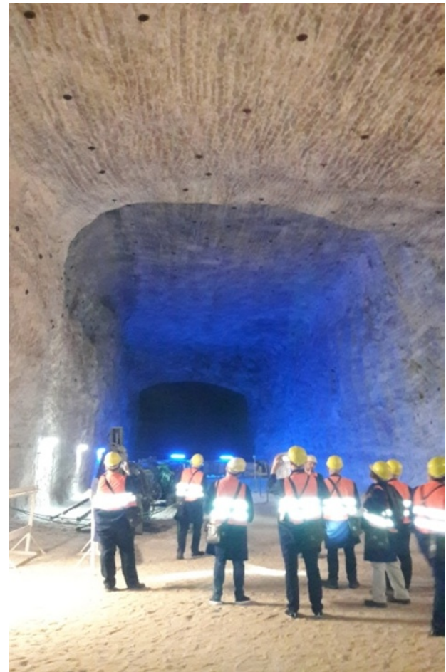
Fig. 3. Room excavation in Kłodawa Salt Mine.
