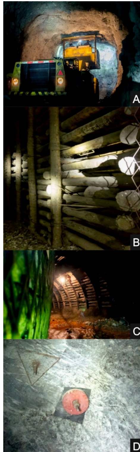
Fig. 2. Additional support of excavations: A) installing of manual rock bolt with steel mesh, B) mining cribs, C) sidewall arch with openwork lagging made by reinforced concrete facing, D) signaling device for roofs stratifications.
