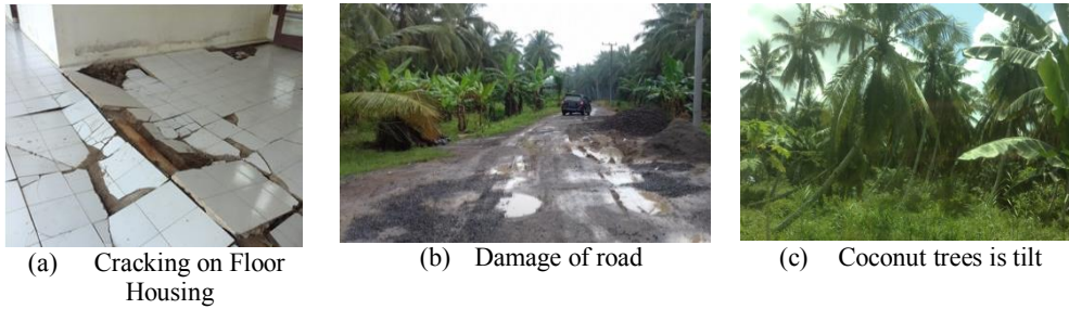
Fig. 4. Direct Impact of Land Subsidence.
