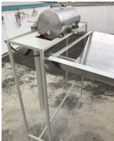
Figure 2. Built in heating system
