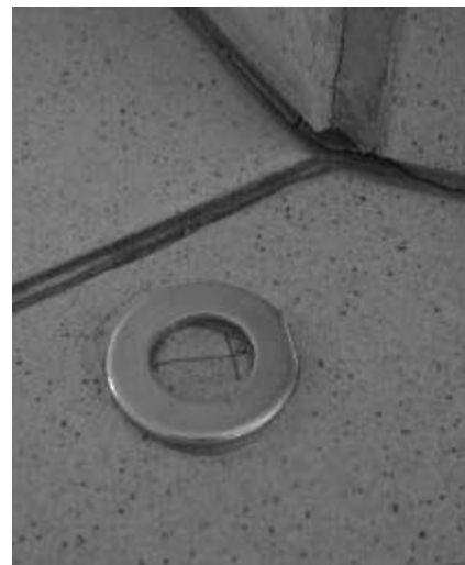
Photo. 3. Stabilisation of the control points on the floor inside the above-ground crossing between buildings.
