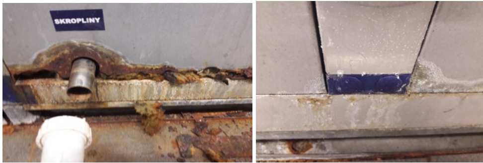
Fig. 1. View of the external cover panels of the air handling unit (air handling unit 1).
