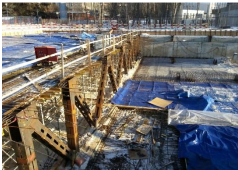
Fig. 5. Construction of 3-storey underground parking. Slab supported by truss structures.
