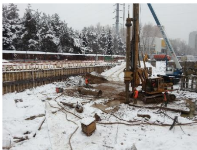
Fig. 2. The retaining structure for the excavation and pile drilling.
