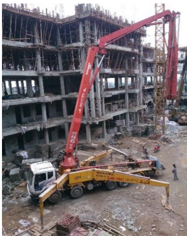
Fig. 1. Pumping concrete mixture through pipelines in the high-rise constructions in Hanoi (Vietnam)
