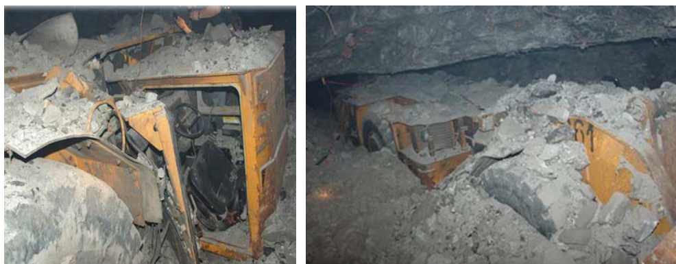
Fig. 2. Damage resulting from the upthrow of machinery caused by a rock burst.
