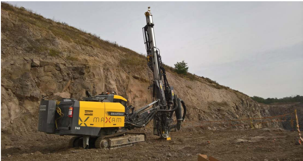
Fig. 1. SmartROC T45 drill rig with a GNSS Leica receiver [7].
