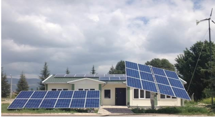
Fig. 1. (a) 12 panels (260 W) with one-axis (right) and without (left) solar tracker platform (b) averaged total daily power generation values of tracking and fixed panels.
