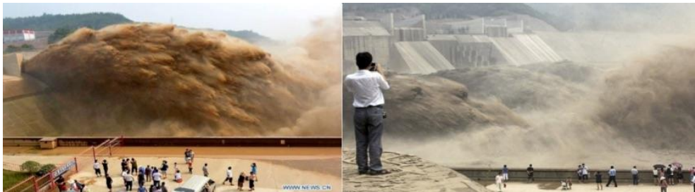
Fig. 5. Clay Mud Discharge at the Xiaolangdi Dam Base in China [15].
