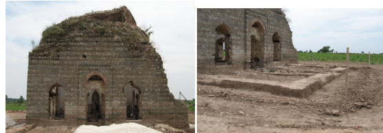
Fig. 2. Photographs before and after restoration of the Timurtaş(Demirtaş) Mosque (2007).
