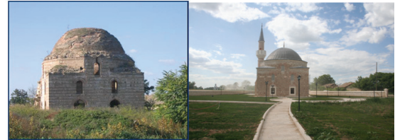
Fig. 1. Photographs before and after restoration of the Timurtaş(Demirtaş) Mosque (2007-2008).
