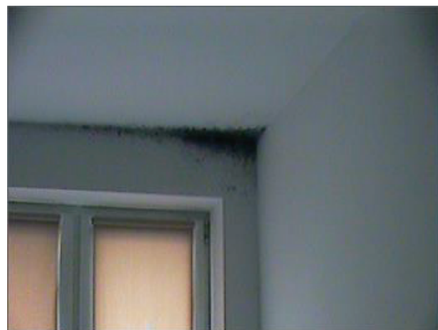
Fig. 7. Detected troubles in the tested residential apartment buildings: mold in the room corner, on the internal surface of the external wall, caused by limited infiltration of external air, poor natural ventilation, thermal bridges and significant moisture gains from people.
