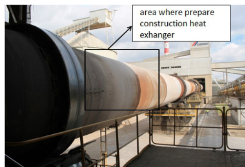
Figure 4. Rotary boiler number 4
