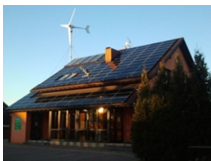
Figure 2. Use of alternative sources of energy: photovoltaic cells and 0.5 kW household wind turbine. “EKOMOTEL na Wierzyńka”. Wieliczka near Krakow (photo by Ł. Steg)
