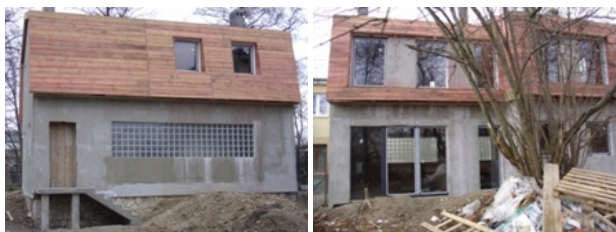
Figure 3. Improperly designed new building. a. south-western façade without glazing, b. northern façade – fully glazed, Kraków, Zarzecz street (photo by: W. Sobczyk)
